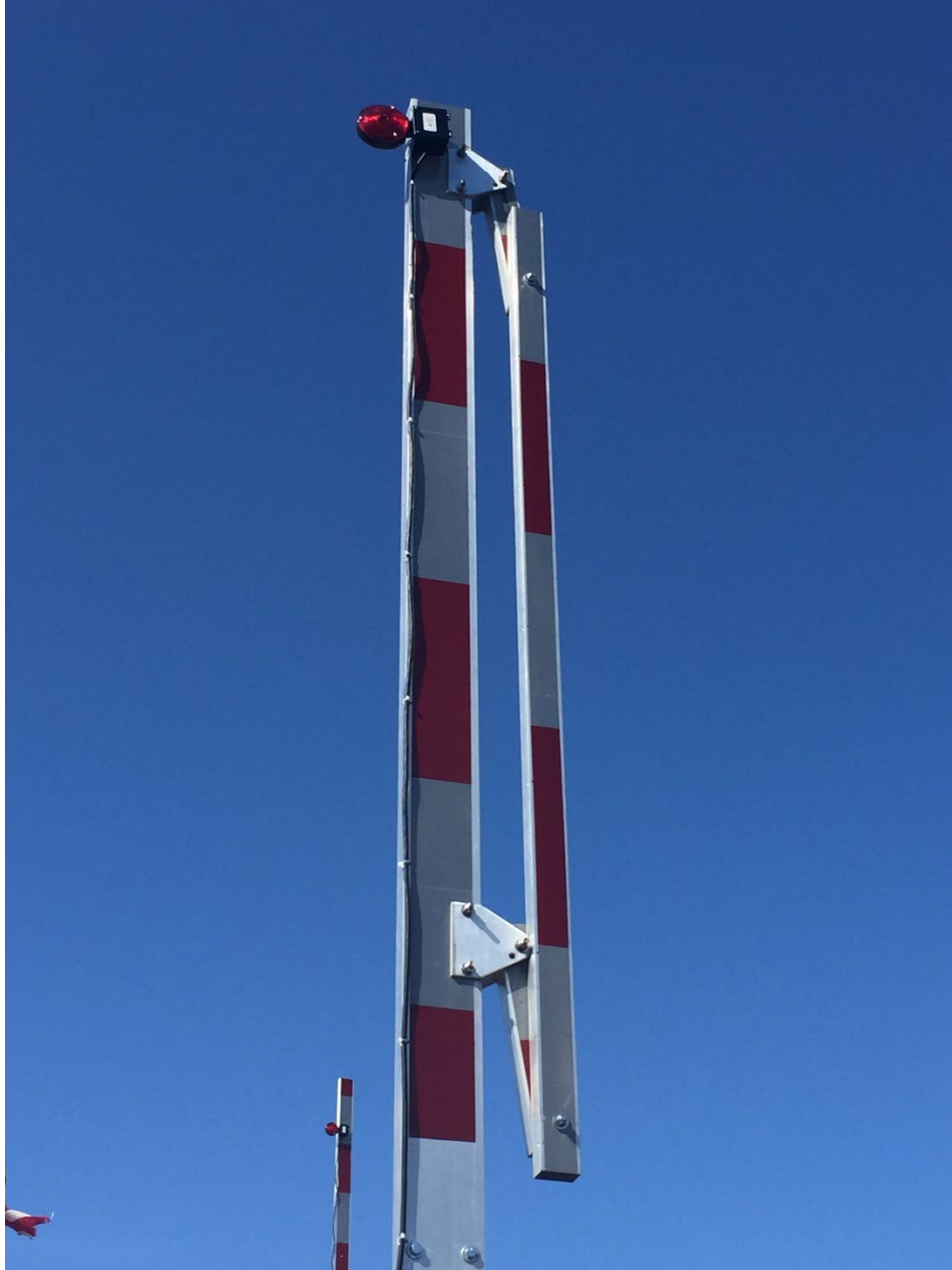
Figure 4. Example of a hinged pedestrian gate skirt in upright position at a grade crossing in Ramsey, NJ Image Credit: Volpe Center
