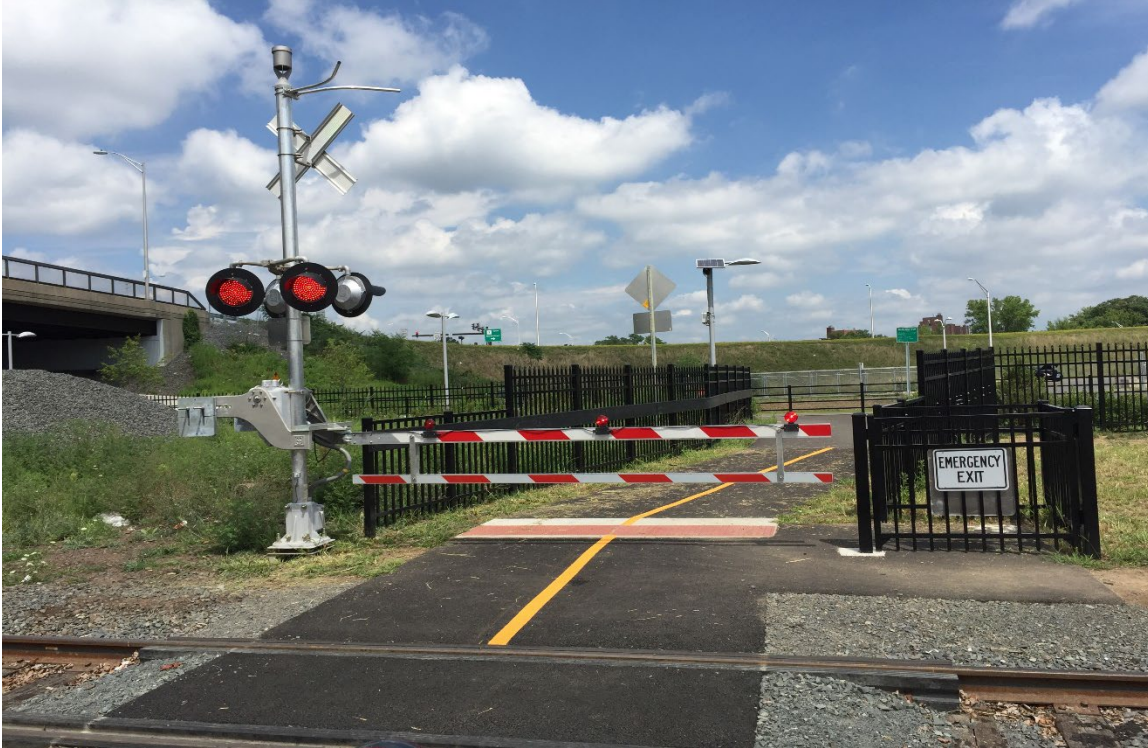
Figure 2. Example of a hinged pedestrian gate skirts at a pathway crossing in New Britain, CT Image Credit: Volpe Center
