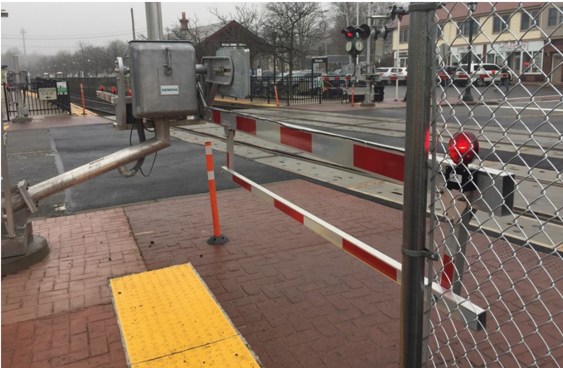
Figure 3. Example of a pedestrian gate skirts with ROW fencing at a grade crossing in Ramsey, NJ Image Credit: Volpe Center
