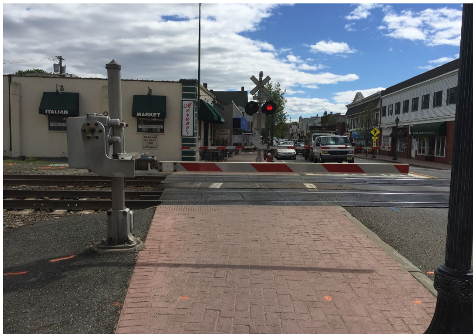
Figure 2. Example of automatic pedestrian gate in Ramsey, NJ Image Credit: Volpe Center
