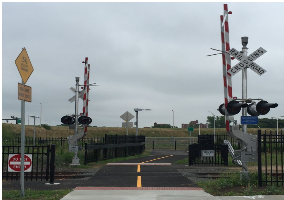
Figure 4. Example of automatic pathway gate with emergency escape gate in New Britain, CT Image Credit: Volpe Center
