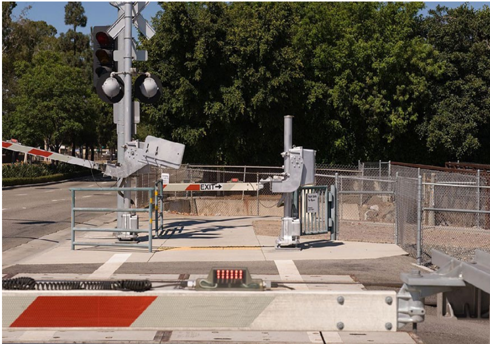
Figure 1. Example of automatic pedestrian gate with emergency escape gate Image Credit: FRA, Grade Crossing Handbook
