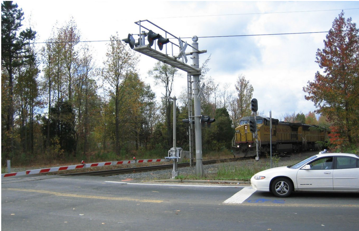
Figure 1. Example of longer arm gate at a grade crossing in Charlotte, NC Image Credit: Volpe Center
