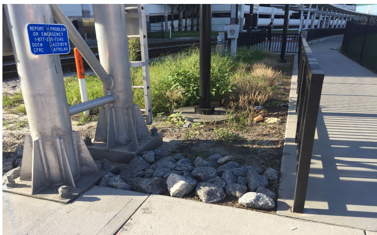
Figure 7. Example of pedestrian channelization using oversized ballast at a grade crossing in Orlando, FL Image Credit: Volpe Center
