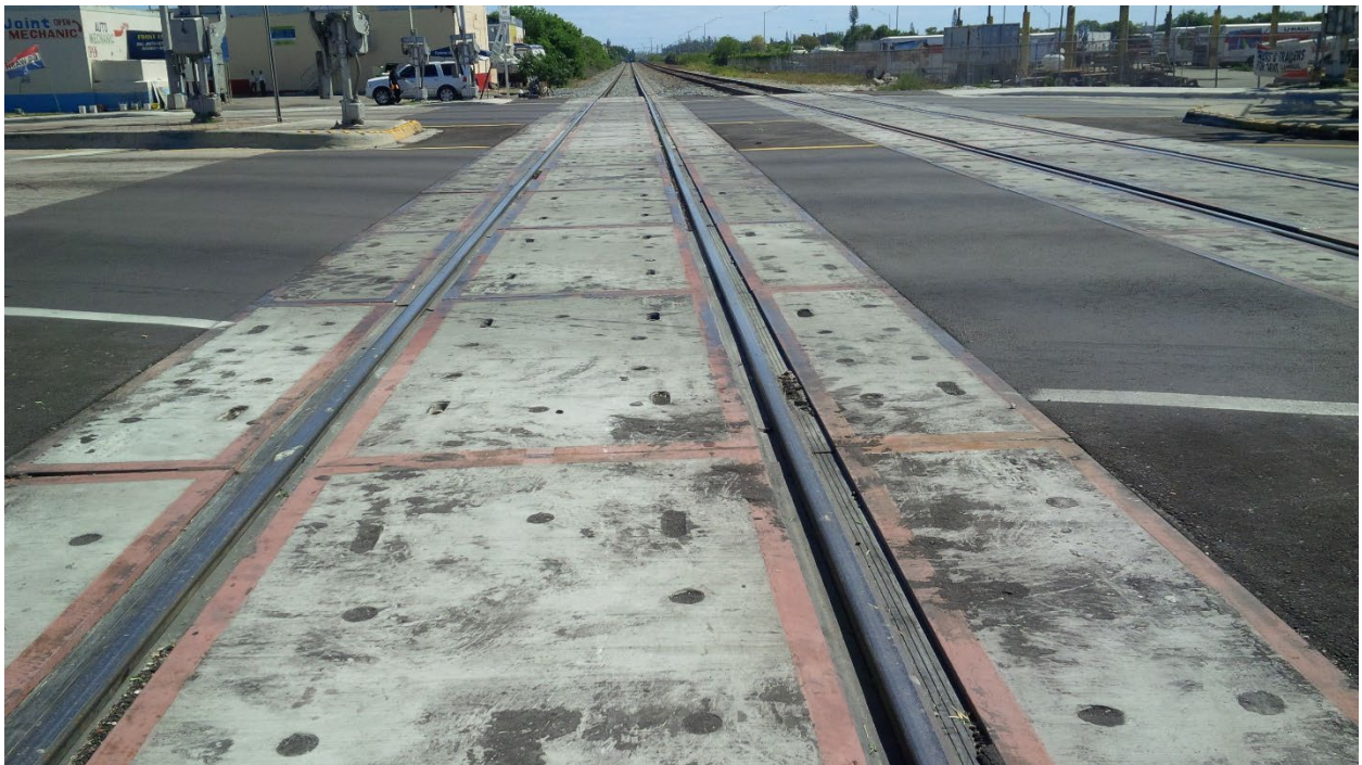
Figure 2. Example of flangeway gap filler at a grade crossing in Opa Locka, FL Image Credit: Volpe Center
