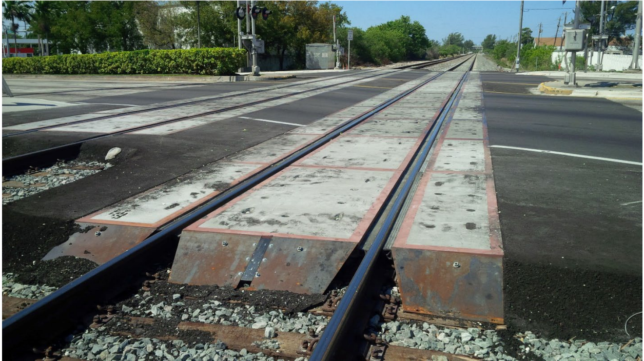
Figure 1. Example of flangeway gap filler at a grade crossing in Opa Locka, FL Image Credit: Volpe Center
