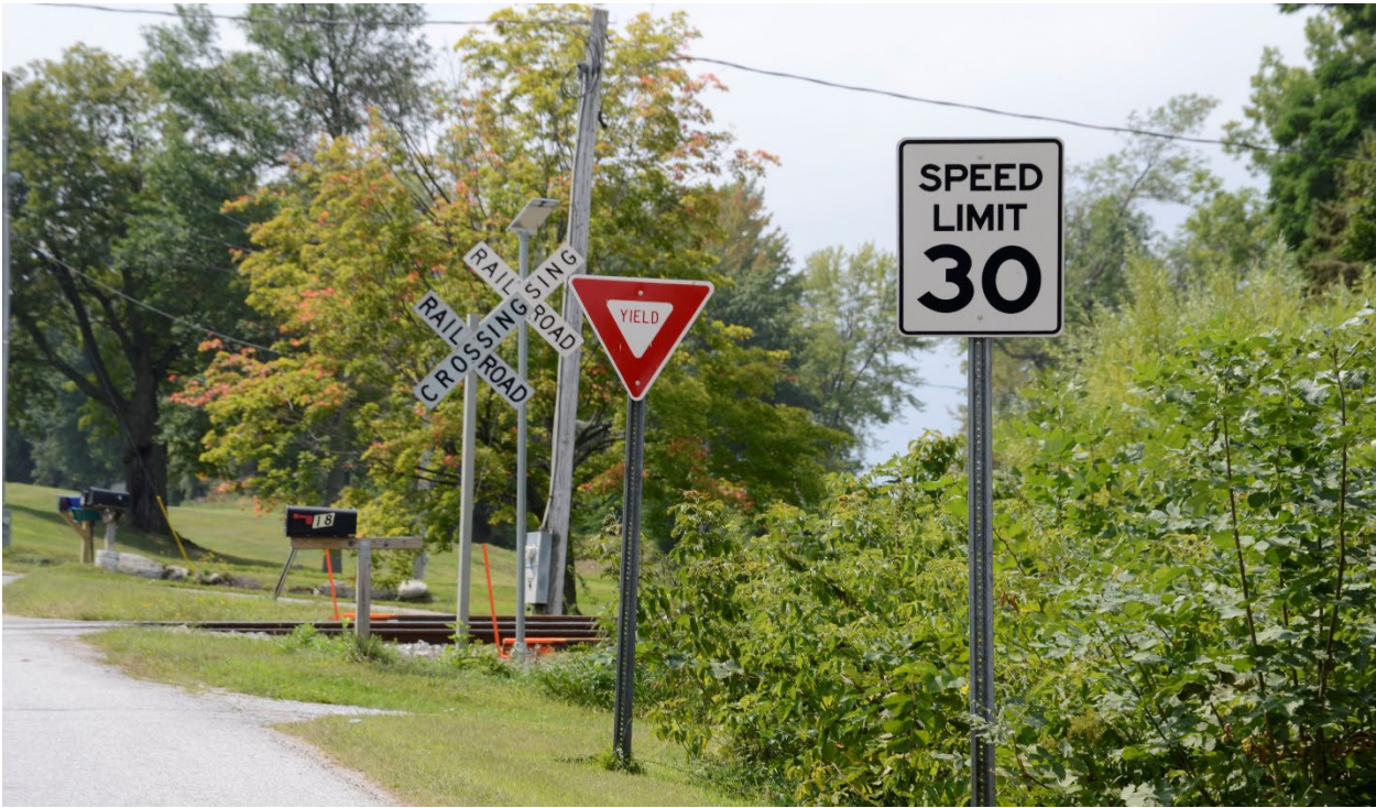
Figure 5. Example of vegetation obstructing pedestrian and driver view of the tracks at a passive crossing in Swanton, VT
