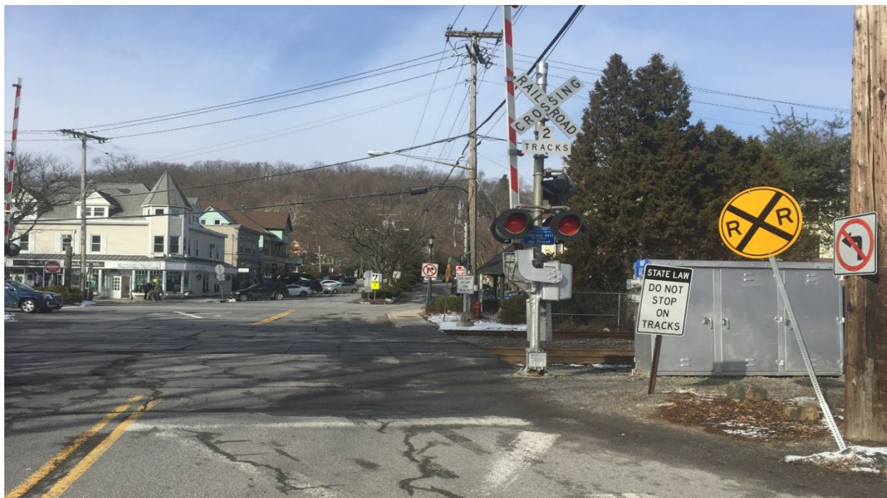
Figure 4. Example of signal cabinet obstructing pedestrian and driver view of the tracks in Katonah, NY Image Credit: Volpe Center
