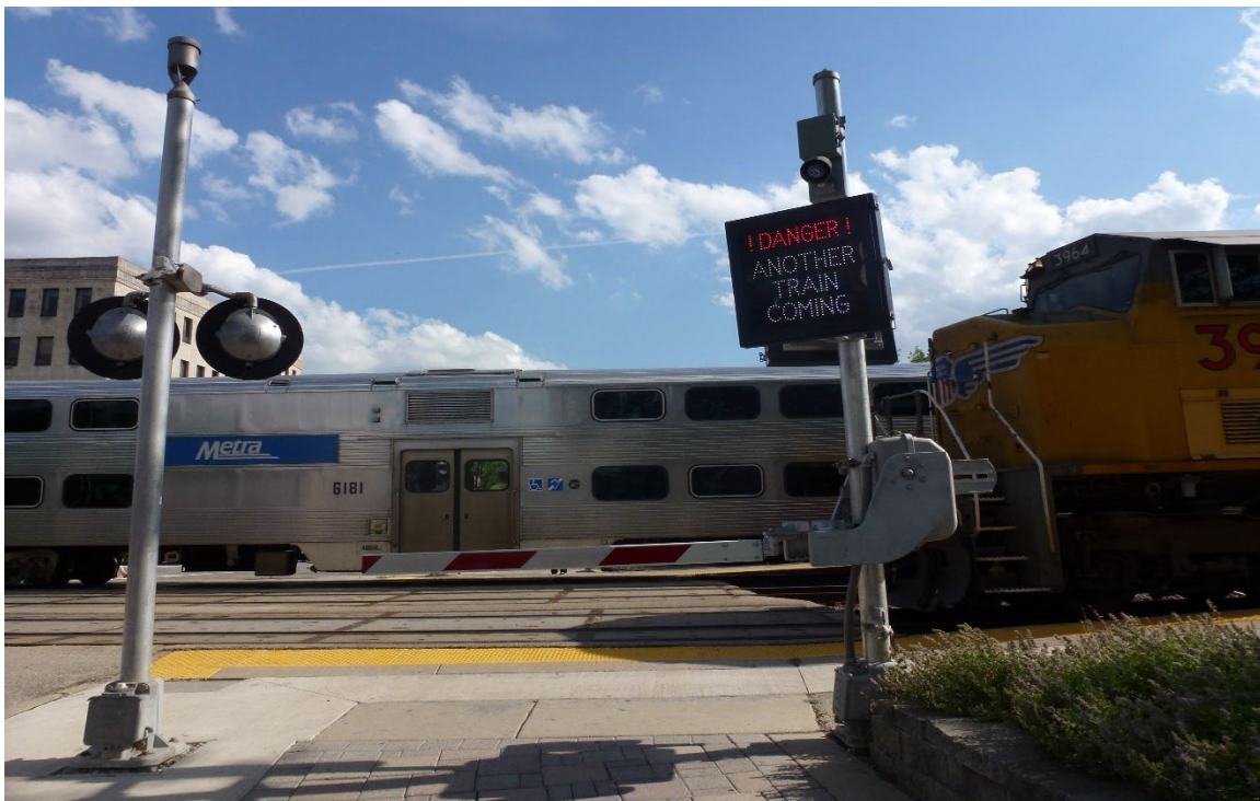
Figure 5. Example of a second train warning system at a crossing in Elmhurst, IL Image Credit: Volpe Center
