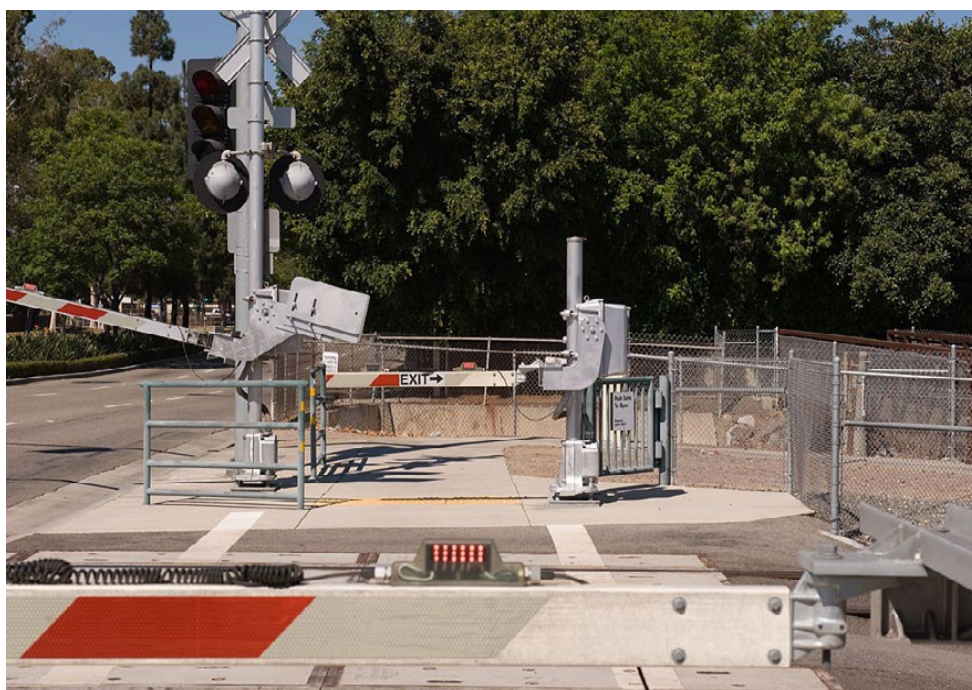
Figure 1. Example of automatic pedestrian gate with emergency escape gate Image Credit: Highway-Rail Crossing Handbook
