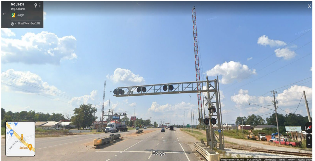
Figure 1. Barrier gates from Google Street View
