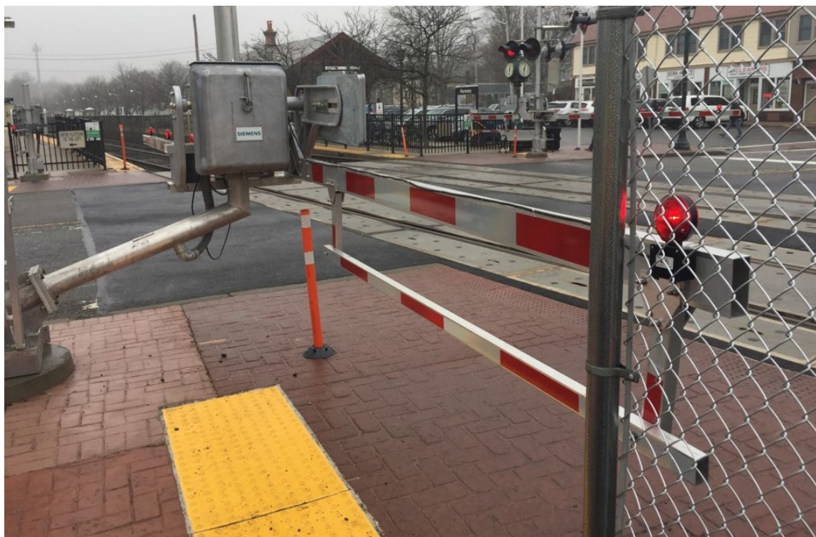
Figure 3. Example of a pedestrian gate skirt with ROW fencing at a grade crossing in Ramsey, NJ Image Credit: Volpe Center
