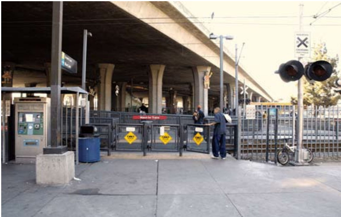
Figure 2. Example of manual swing gate Image Credit: FRA, Compilation of Pedestrian Safety Devices In Use at Grade Crossings
