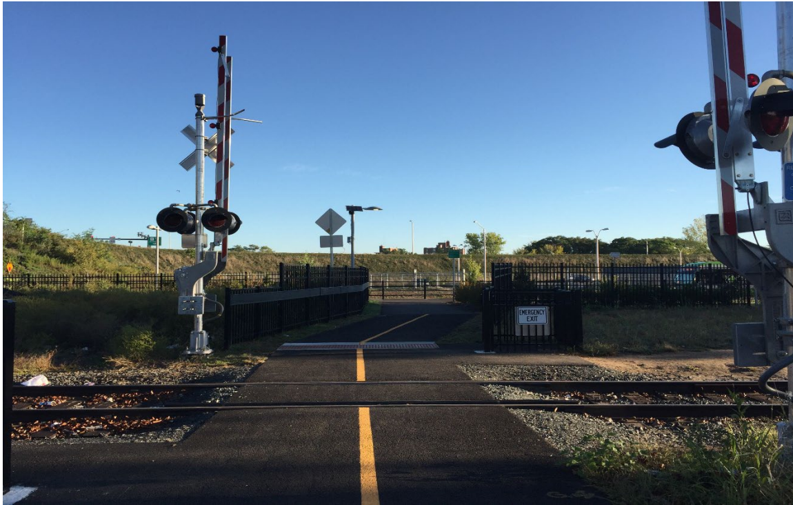
Figure 1. Example of manual swing gate at a pathway crossing in New Britain, CT Image Credit: Volpe Center
