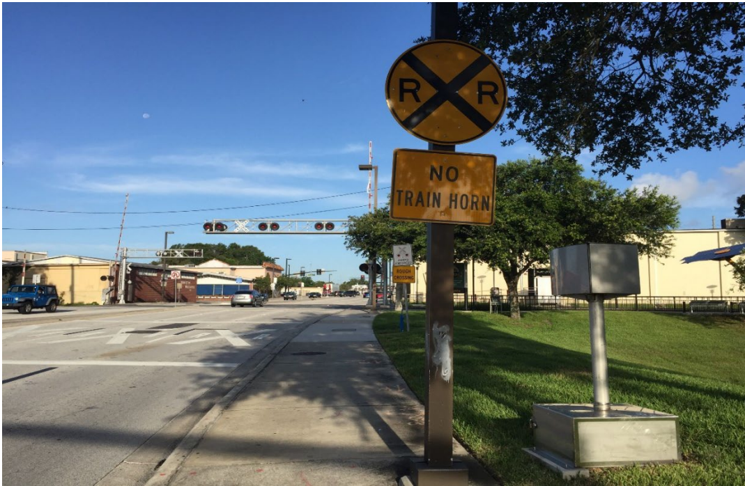
Figure 1. Photo enforcement system at a grade crossing in Orlando, FL Image Credit: Volpe Center
