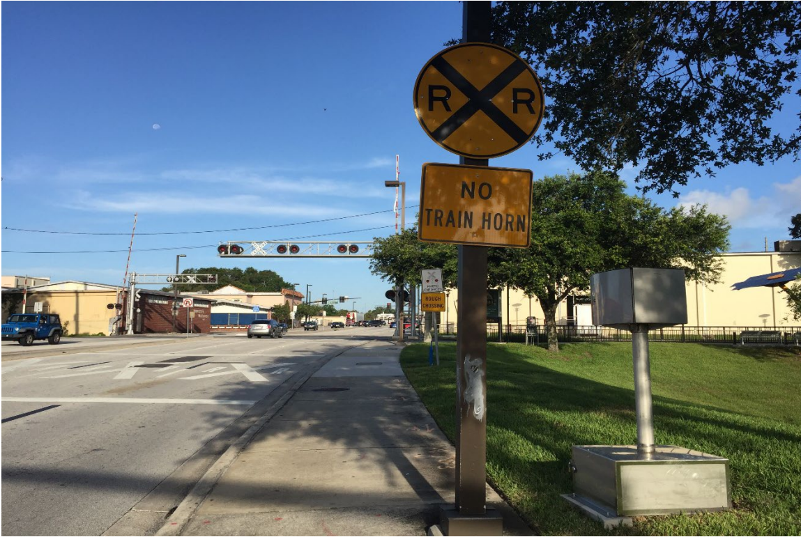
Figure 1. Photo enforcement system at a grade crossing in Orlando, FL Image Credit: Volpe Center
