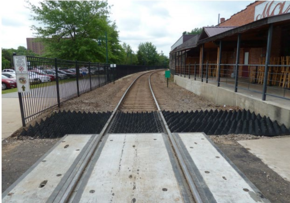
Figure 1. Anti-trespass panels installed at a grade crossing in Fayetteville, AR. Image Credit: Volpe Center
