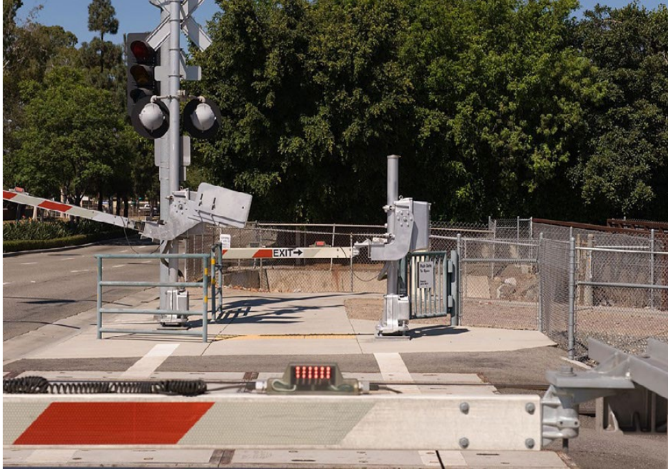
Figure 2. Example of automatic pedestrian gate with emergency escape gate. Image Credit: FRA, Grade Crossing Handbook
