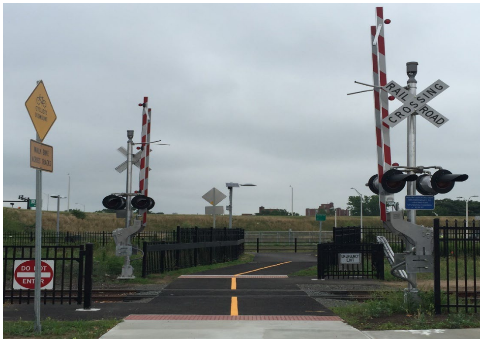
Figure 1. Example of automatic pathway gate with emergency escape gate in New Britain, CT Image Credit: Volpe Center
