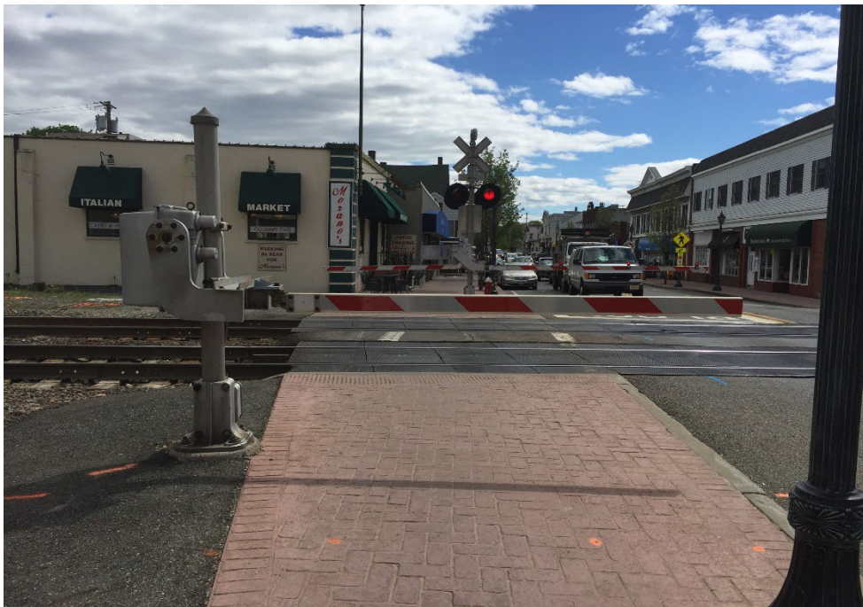
Figure 3. Example of automatic pedestrian gate in Ramsey, NJ Image Credit: Volpe Center
