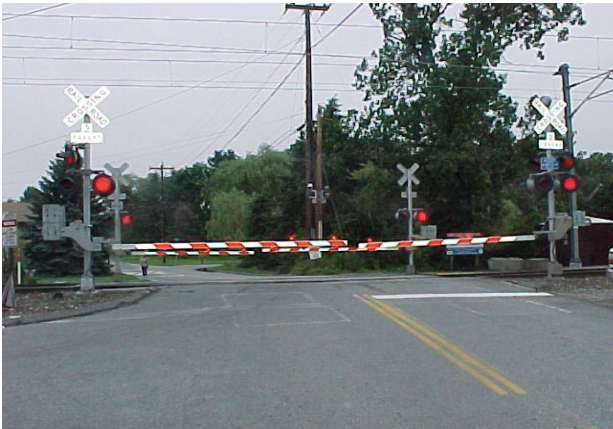
Figure 3. Example of four quadrant crossing gates at a grade crossing in Groton, CT Image Credit: Volpe Center
