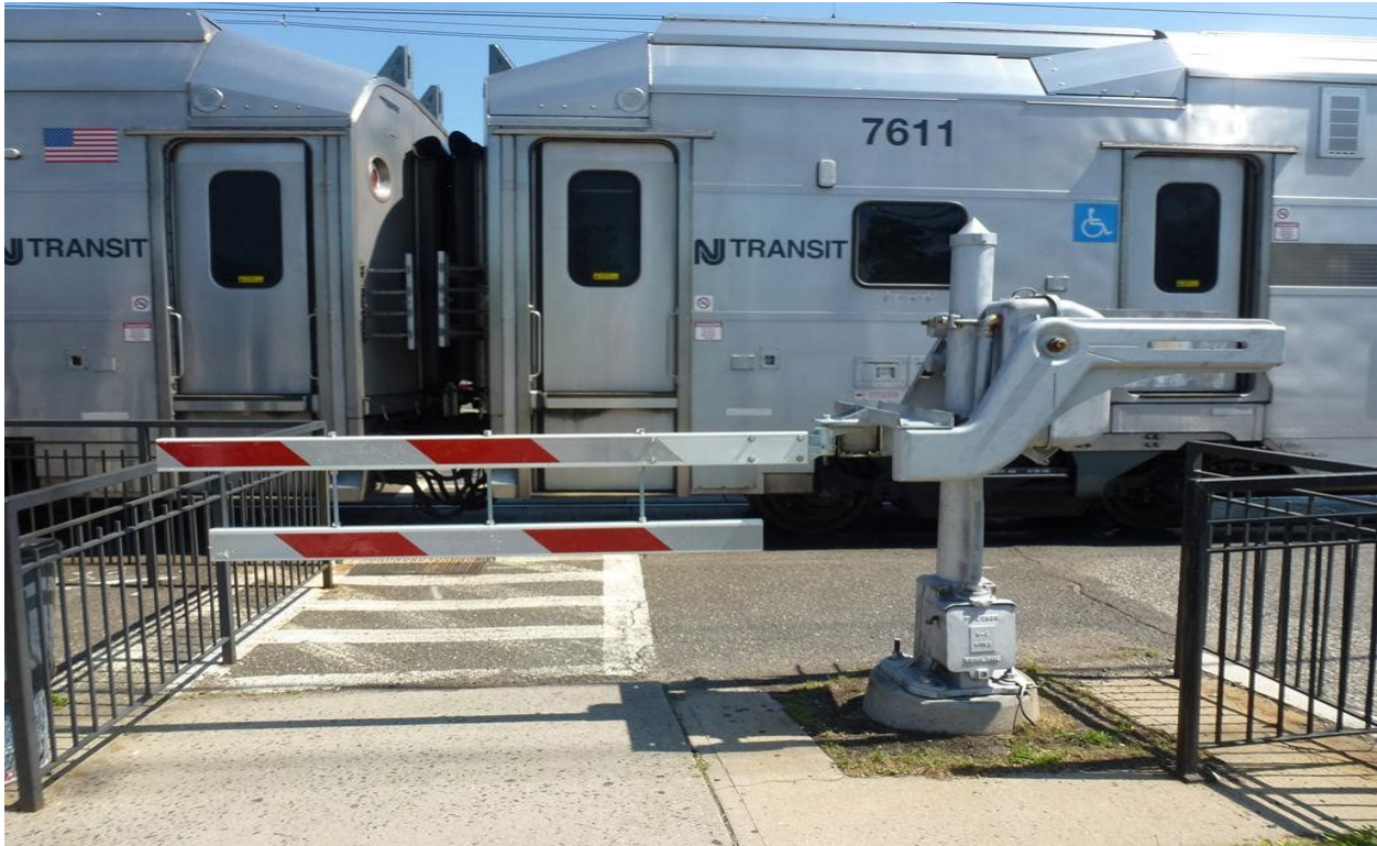
Figure 1. Example of a pedestrian gate skirts with sidewalk fencing at a grade crossing in Matawan, NJ Image Credit: Volpe Center
