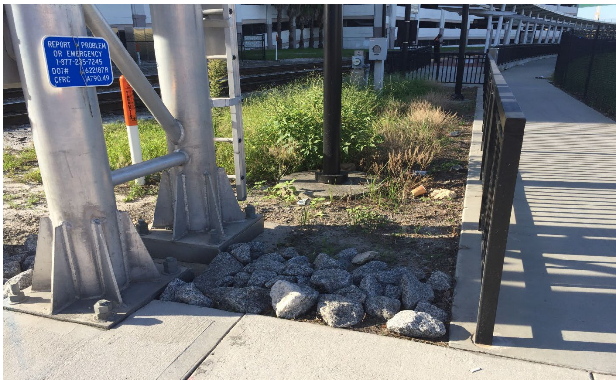
Figure 7. Example of pedestrian channelization using oversized ballast at a grade crossing in Orlando, FL Image Credit: Volpe Center
