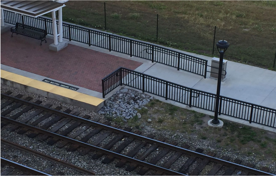
Figure 3. Rock treatments to prevent commuters from using ROW as a shortcut between station and crossing. Image Credit: Volpe Center
