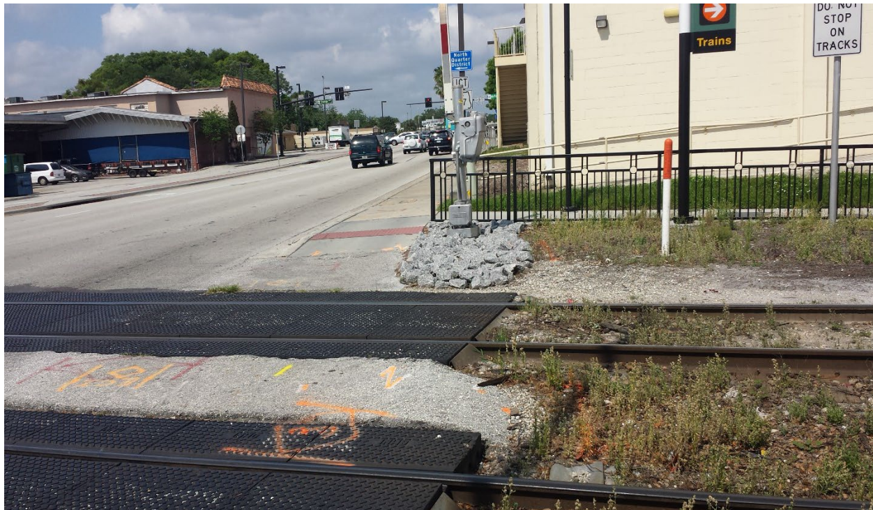
Figure 2. Example of rock treatments at a grade crossing in Orlando, FL Image Credit: Volpe Center
