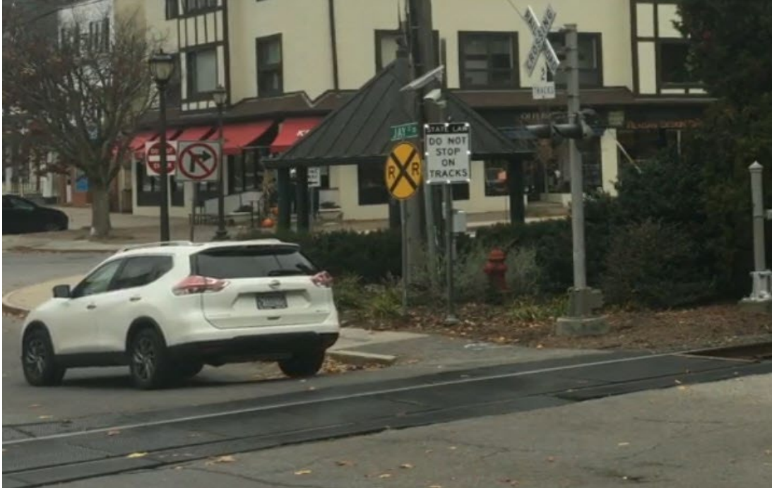
Figure 4. Example of LED-enhanced DO NOT STOP ON TRACKS sign (NYR9-5) at a grade crossing in Katonah, NY Image Credit: Volpe Center
