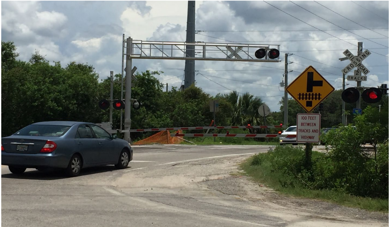
Figure 3. Example of vegetation obstructing pedestrian and driver view of the tracks at a crossing in Osceola County, FL Image Credit: Volpe Center
