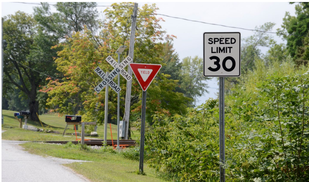
Figure 5. Example of vegetation obstructing pedestrian and driver view of the tracks at a passive crossing in Swanton, VT Image Credit: Volpe Center
