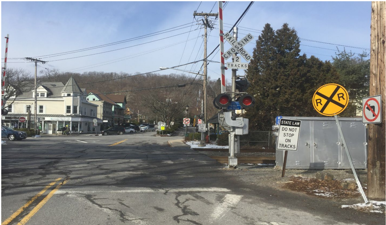
Figure 4. Example of signal cabinet obstructing pedestrian and driver view of the tracks in Katonah, NY Image Credit: Volpe Center
