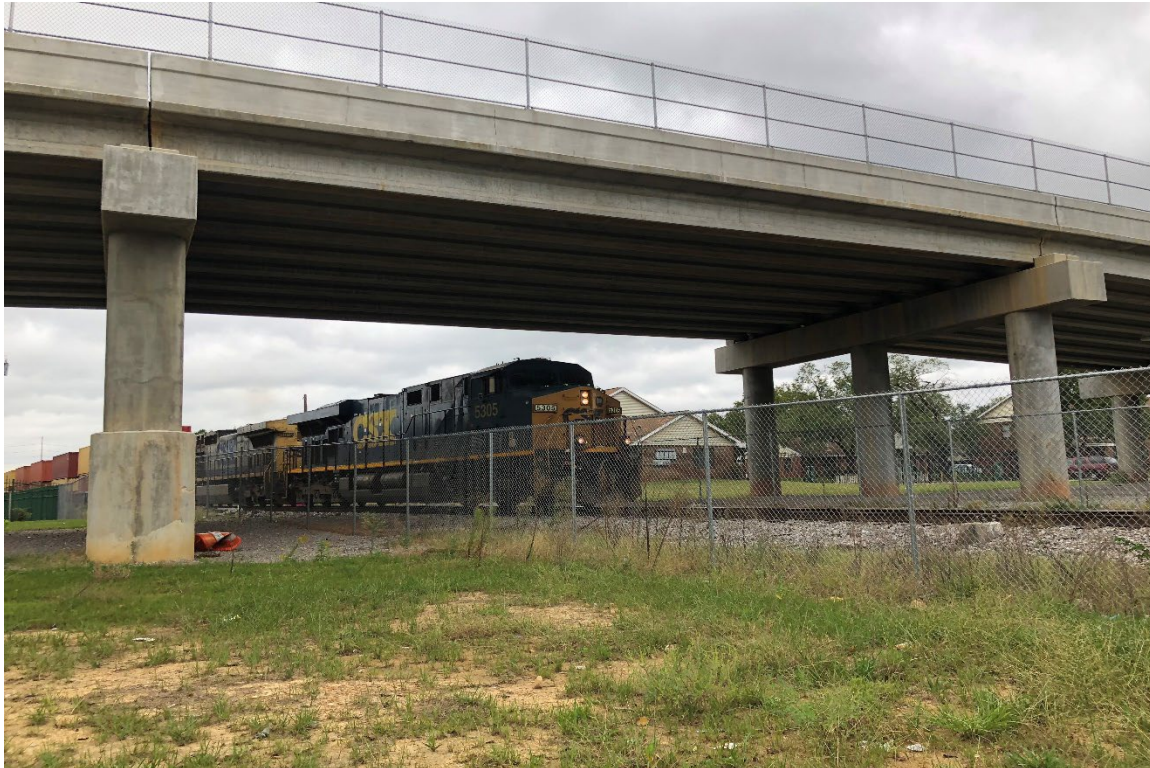
Figure 1. Example of a grade separated crossing in Birmingham, AL Image Credit: Volpe Center
