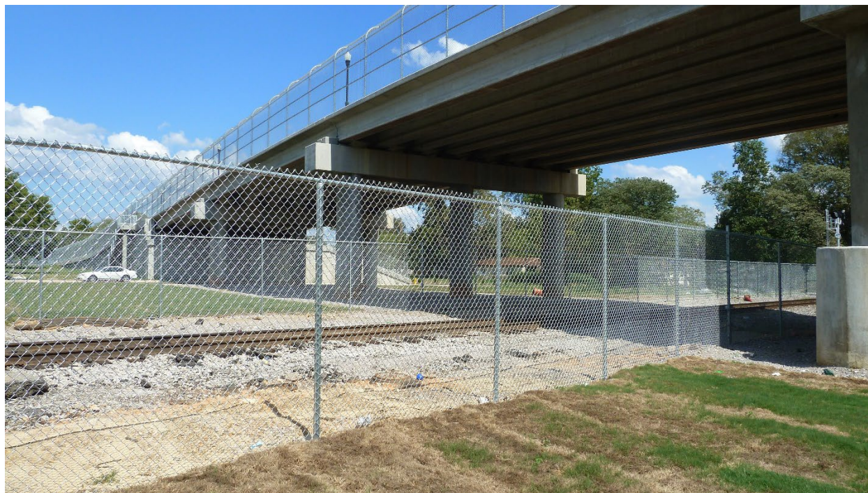
Figure 2. Example of a grade separated crossing in Birmingham, AL Image Credit: Volpe Center
