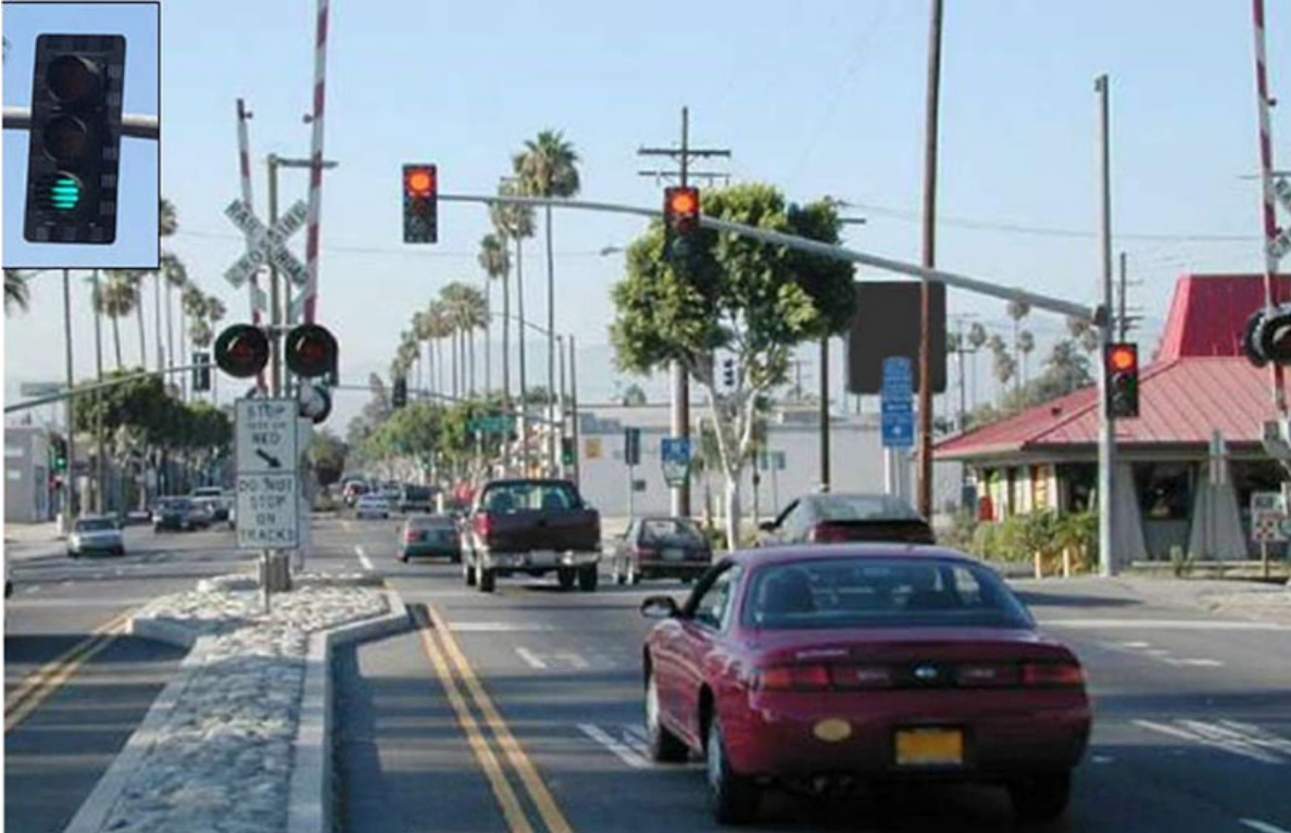
Figure 1. Example of downstream mounted pre-signal at a grade crossing in Fontana, CA Image Credit: FRA, Highway-Rail Crossing Handbook – Third Edition
